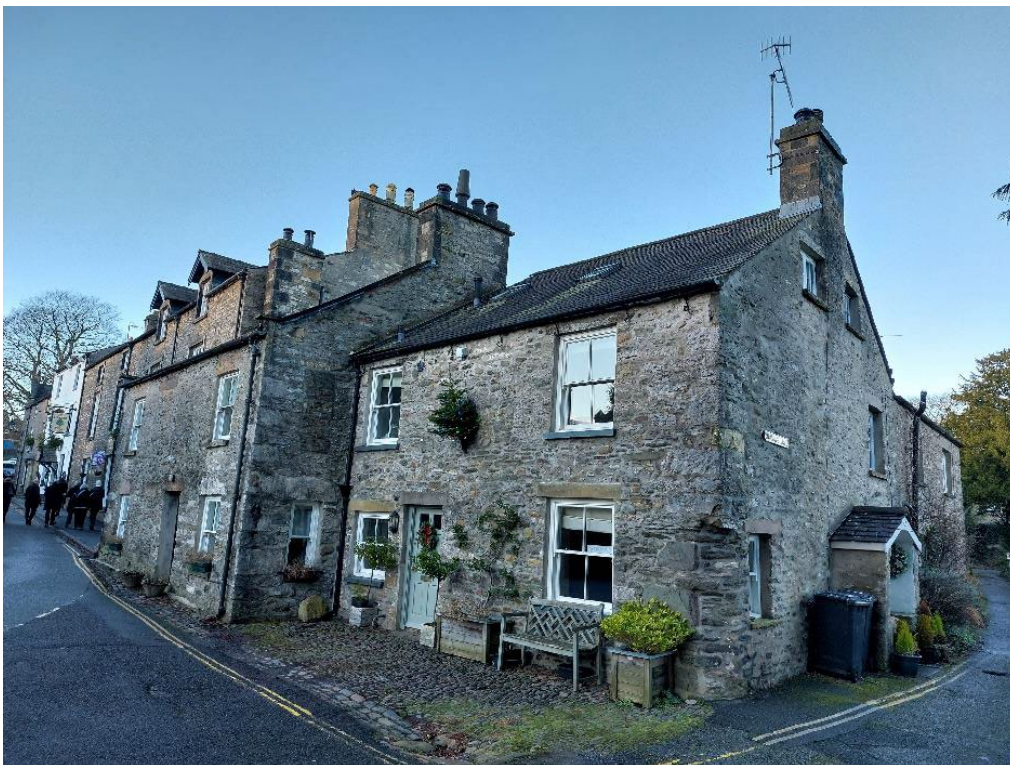
L-shaped terrace with active frontages. It has a range of building heights, set backs and plot widths, but united by the use of gabled forms, traditional proportions and materials. Kirkby Lonsdale.
