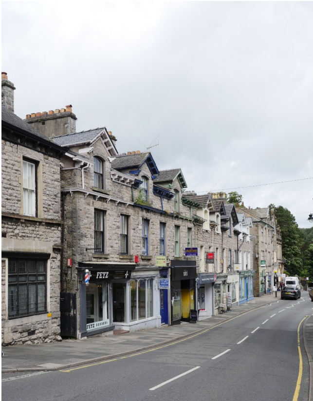
Fine grain, walkable, vibrant settlement with access to shops and services. Grange-over-Sands.
