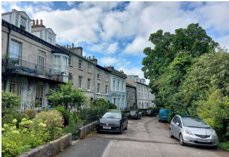
Informal residential street with shared surface and simple speed control. Kendal.
