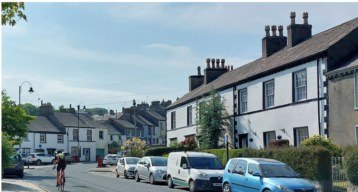
Eaves levels and roof ridges are stepped up the hill. Dalton.
