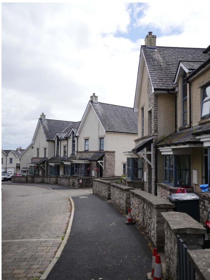
Simple, but solid-looking stone walls echo both the building line and the kerbline and provide a decisive break between private land and the public realm. Grange-over-Sands.
