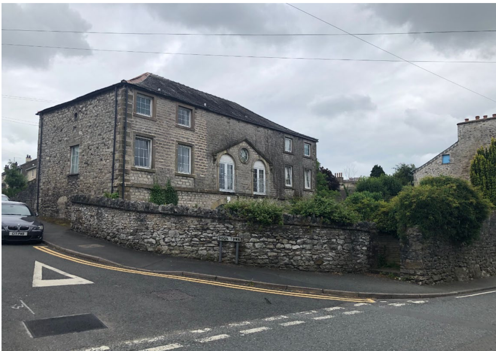
Diminishing rubble courses and rocky coping reinforcing village character. Burton-in-Kendal.
