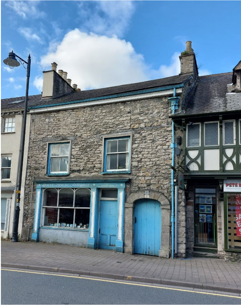
Bare stone walls with timber door and window frames. Kendal
