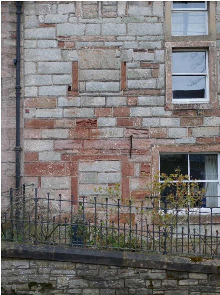
Formal wall and railings giving an urban character. Appleby.
