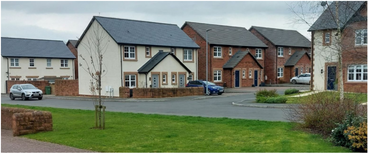
This simple 90-degree T-junction with narrow carriageways means no one is likely to turn the corner at speed, making a safer and more inviting street. Temple Sowerby.
