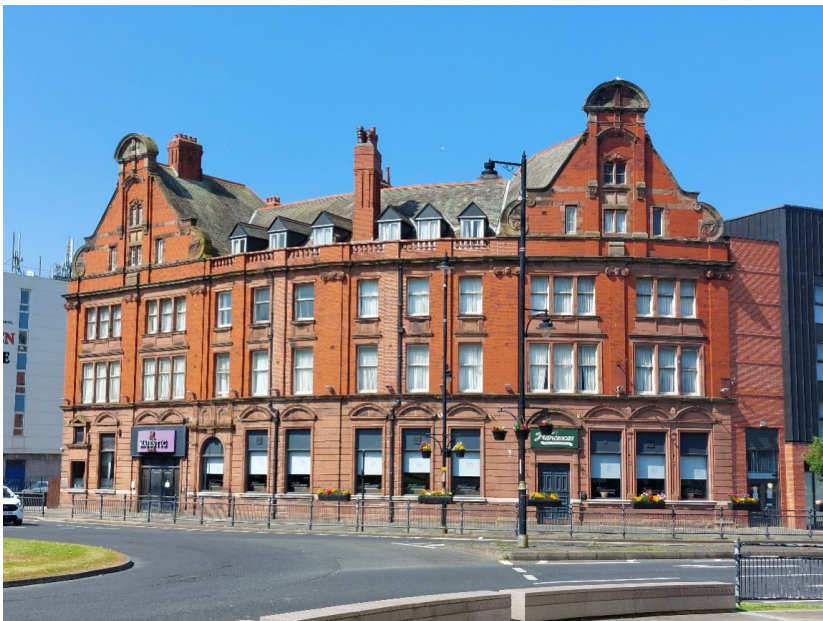
Red brick is a common material in specific areas, seen on houses, commercial buildings, walls and chimneys. Barrow.
