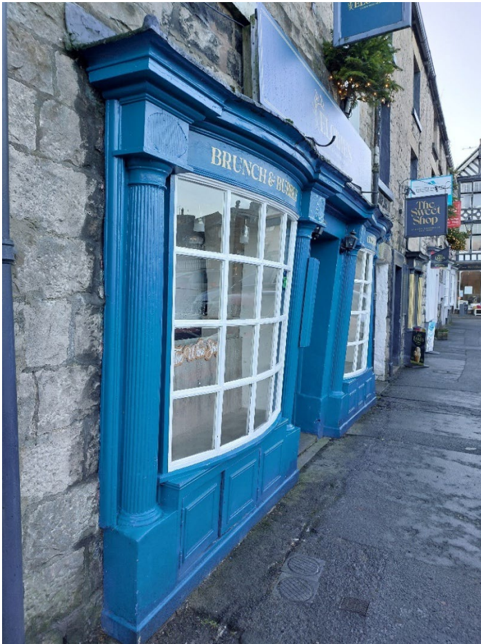
Timber shop fronts set within exposed, coursed stone walls. Kirkby Lonsdale.
