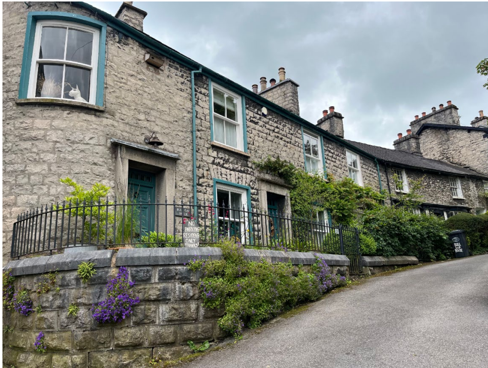
Retaining wall and railing creating a two-tier boundary that assists with creating a level access on sloping land. Kendal.
