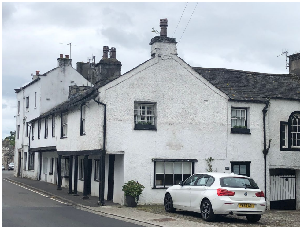
Phases of development seen from street level. Burton-in-Kendal.
