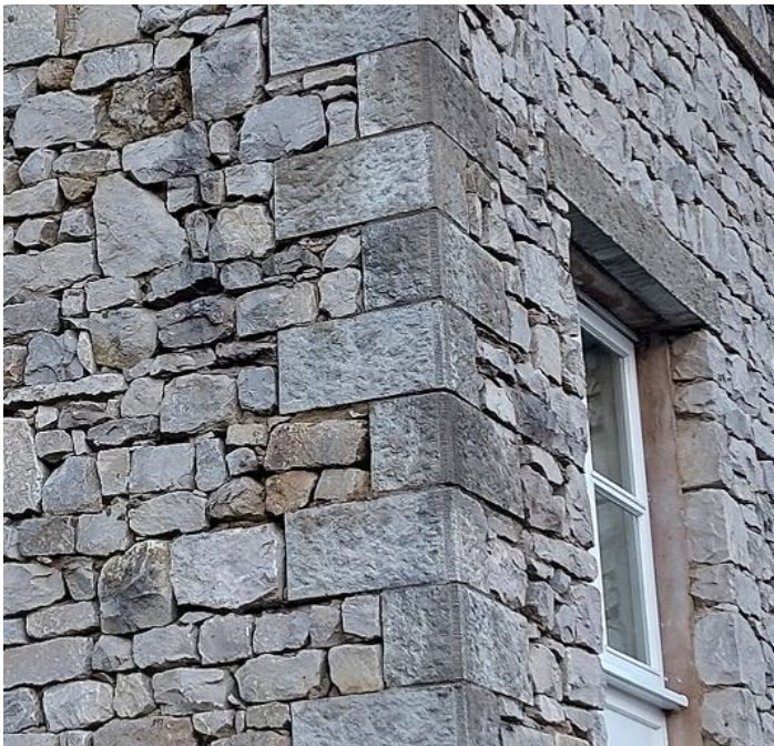
This newbuild in Kirkby Lonsdale makes excellent use of stone for walling quoins (or cornerstones) and sills and lintels. The thickness of the walls shelters the timber windows and give the building a sturdy and vernacular character.
