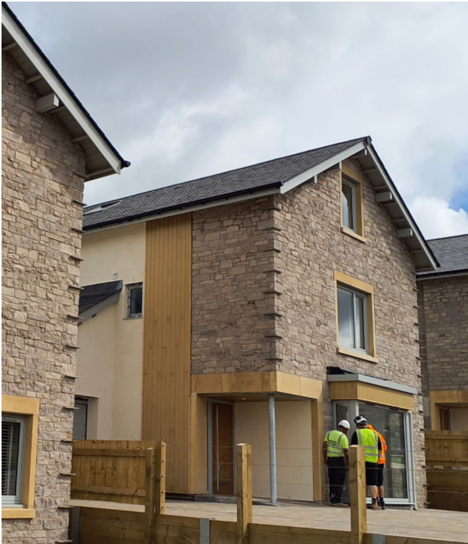
A contemporary material hierarchy using stone, timber cladding and roughcast render, with smooth reveals for the openings. Lindal-in-Furness.
