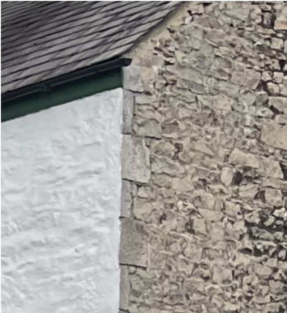
Even on humbler buildings like cottages, the painting of the stonework on the front elevation (left) gives a cleaner and neater appearance than the underlying bare rubble on the side elevation (right). Kendal.
