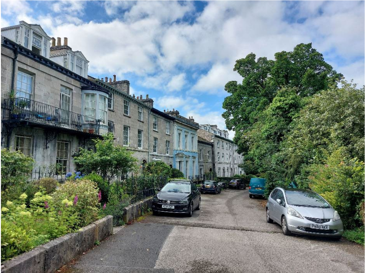
Although this development predates cars, the simplicity of the shared surface and informal provision of parking makes the space very uncluttered. Kendal.
