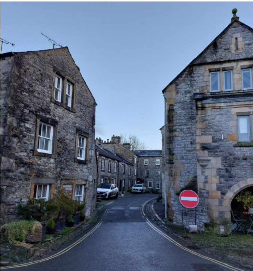
Terraces are common, but the buildings within them have different heights and widths. Parking is informal and in front of the houses. The intimate built form and closeness of the buildings at the entrance to the street give it an enclosed courtyard feel. Kirkby Lonsdale.
