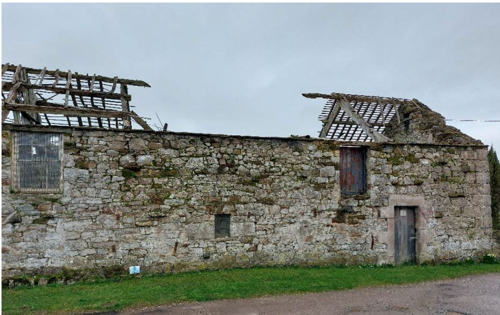
Although derelict, the walls of this barn at Stainton near Penrith are embodied carbon that may be capable of repair, re-use or as a last resort, a source of recycled materials.
