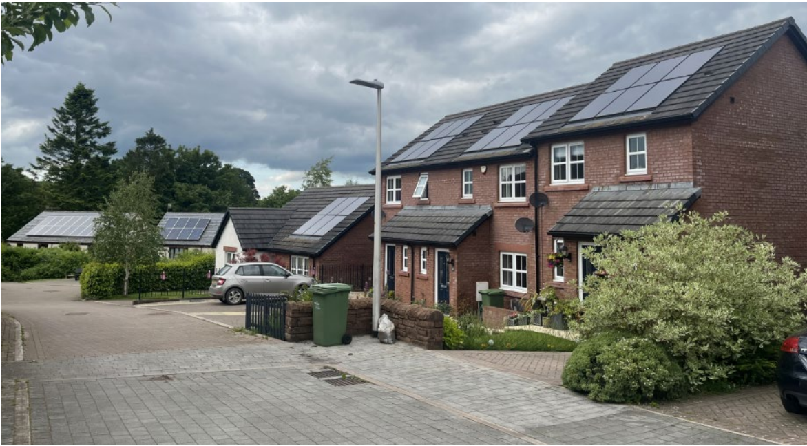
PV panels have been built into the roof slopes in the foreground when these houses were built, meaning the surfaces of the panels are almost flush with the roof tiles. In the background PV panels have been retrofitted to existing slate roofs. Lazonby.
