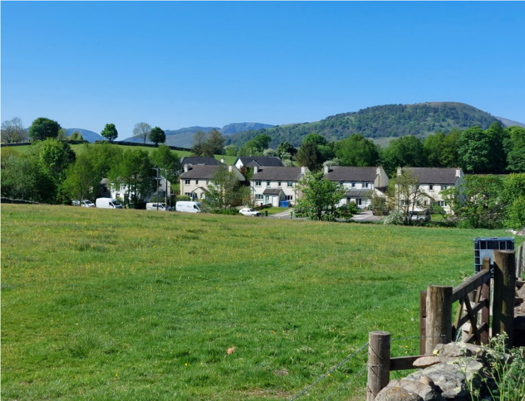
This row of houses in Motherby has a clear building line. The roof ridges, eaves, and elevations all form a straight line from left to right.
