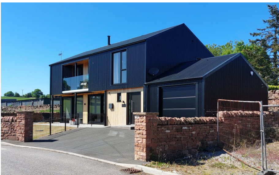
This new house in Great Salkeld has its principal rooms facing south to maximise solar gain. Overheating is managed by the recessing of the glazing and internal blinds.
