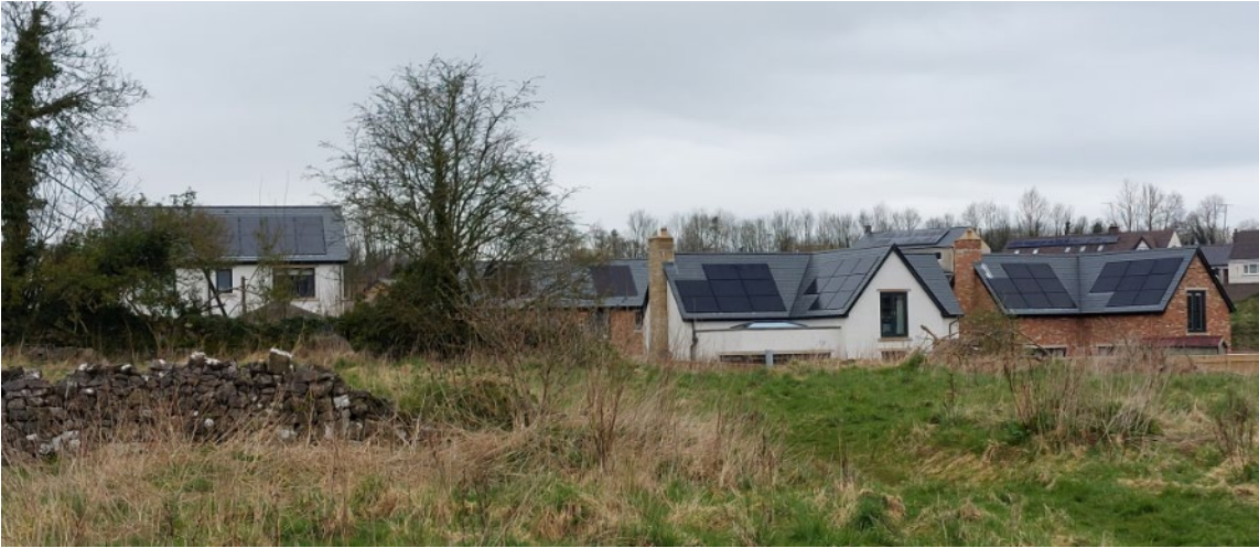
This housing development in Stainton near Penrith makes extensive use of solar panels on the southerly facing roof pitches. The panels are set into the roof slopes.
