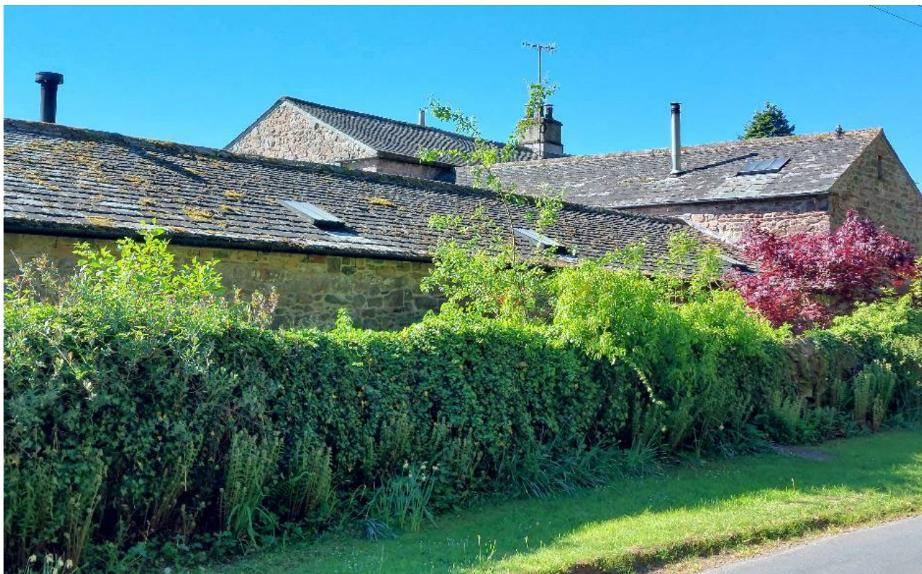
These two converted barns retain traditional uninterrupted roofs. The few rooflights and flues are the only indication from the street of the conversions. Greystoke.
