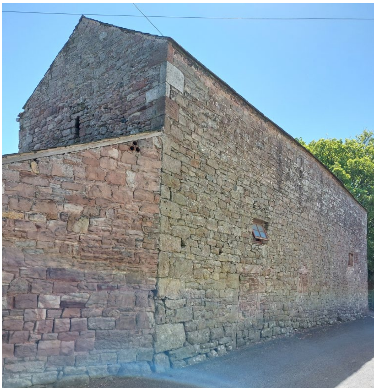
Here the stonework provides clues of the building's development: the differences in stone on the long elevation show the height of the barn was raised in the past, the pinker stone of the lean-to show this was a later addition, while there are signs of a filled in door and window on the long elevation. Skelton.
