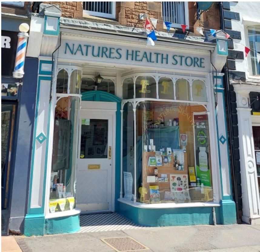
This shopfront in Penrith has a degree of shade and shelter provided by the cornice and recessed doorway. The awning just above the shop sign (with iron arms at either end) provides an excellent way of stopping the inside of the shop from overheating in strong sunlight, as well as providing shelter for customers
