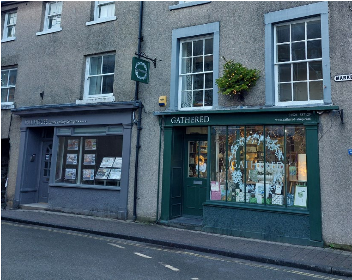
Two shopfronts in Kirkby Lonsdale. Different heights and slightly different proportions and details, but the components used and the depth and shadow they create are the same.
