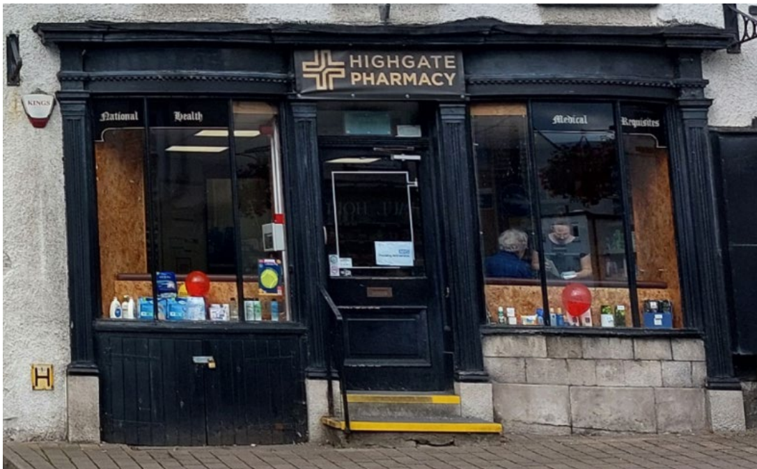
Levelled steps, contrasting step edges and a handrail are all reasonable adjustments to this late Georgian shopfront in Kendal.
