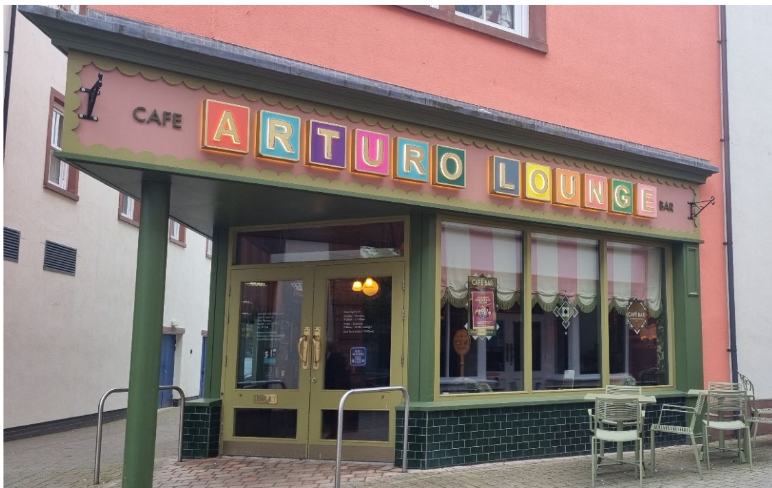
At this modern building in Penrith, the shopfront has a range of projecting and recessed features giving it depth and shadow. The corner doorway is set back from the building line, creating a sheltered and recessed entrance to the business.
