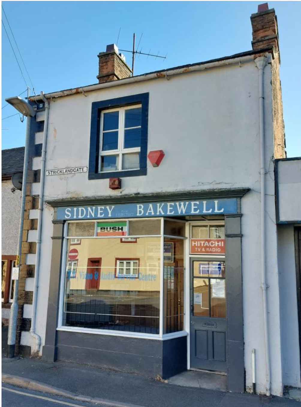
A simple but well-proportioned shopfront on a side street in Penrith town centre. It appears to be a late Georgian building and shopfront, but the white frames and door are perhaps from the mid-20th century. A shopfront can be attractive without being intricate or grand. The proportions and projections and recesses are what brings it to life.
