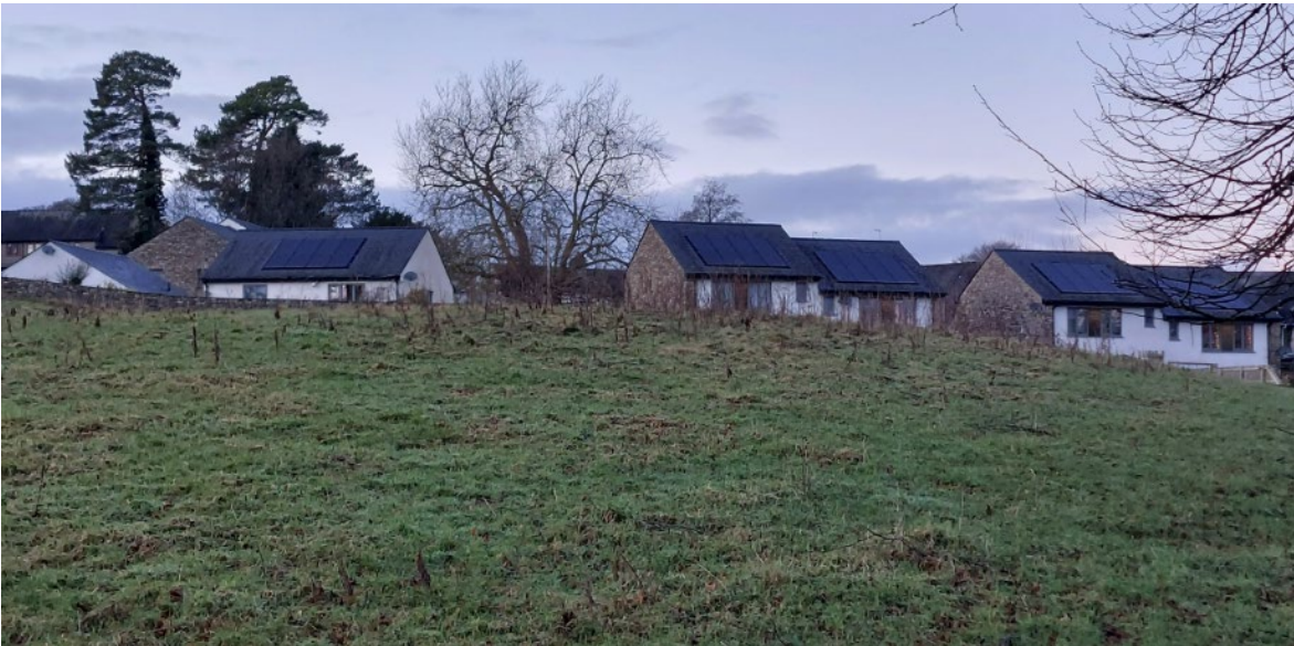
These solar panels blend well with the natural slate of the roofs. The slates form thick borders around the panels, which are placed centrally on the roof slopes. Kirkby Lonsdale.
