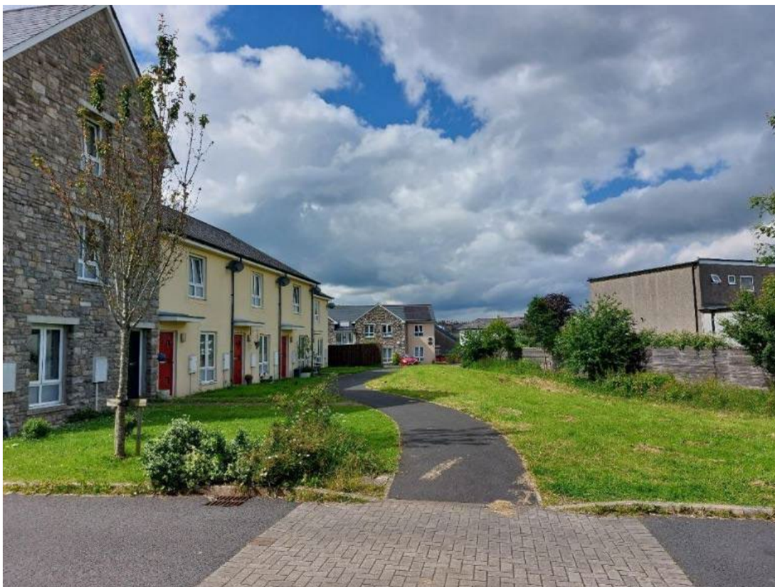
This small piece of green infrastructure near Kendal town centre provides a shortcut between streets, access to houses, visual amenity and space for informal play, and is a component of the site's SuDS, absorbing runoff and draining it away from buildings. A more species rich planting scheme could enhance its ecological value.
