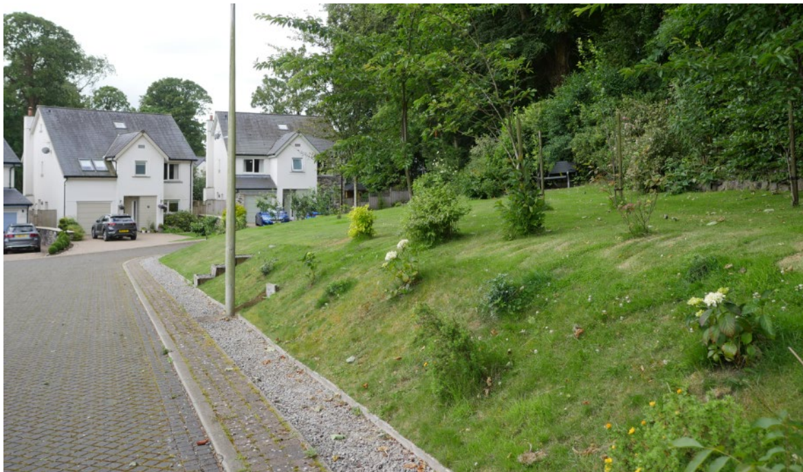
Where the houses are in a lower part of the site, a combination of soft landscaping, a gravel drainage channel and permeable highway surfaces have been used to intercept rainfall and runoff from higher up. Ulverston.
