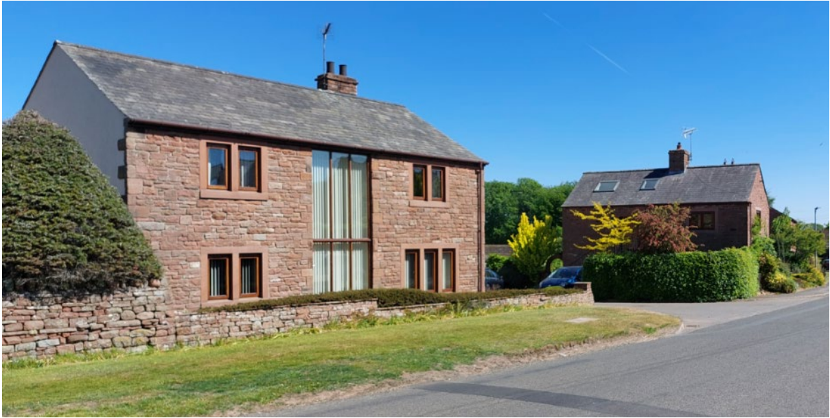
A shared drive that places cars behind the building line and gardens upholds the village character of Great Salkeld.
