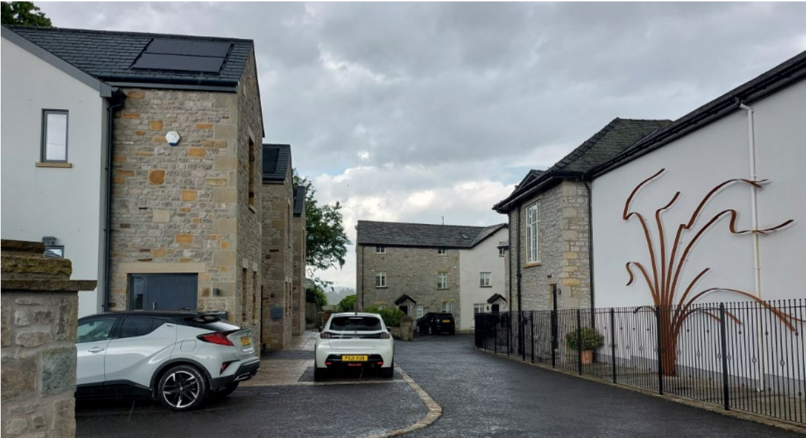
These solar water heaters sit neatly and unobtrusively on these roofs in Kirkby Lonsdale.
