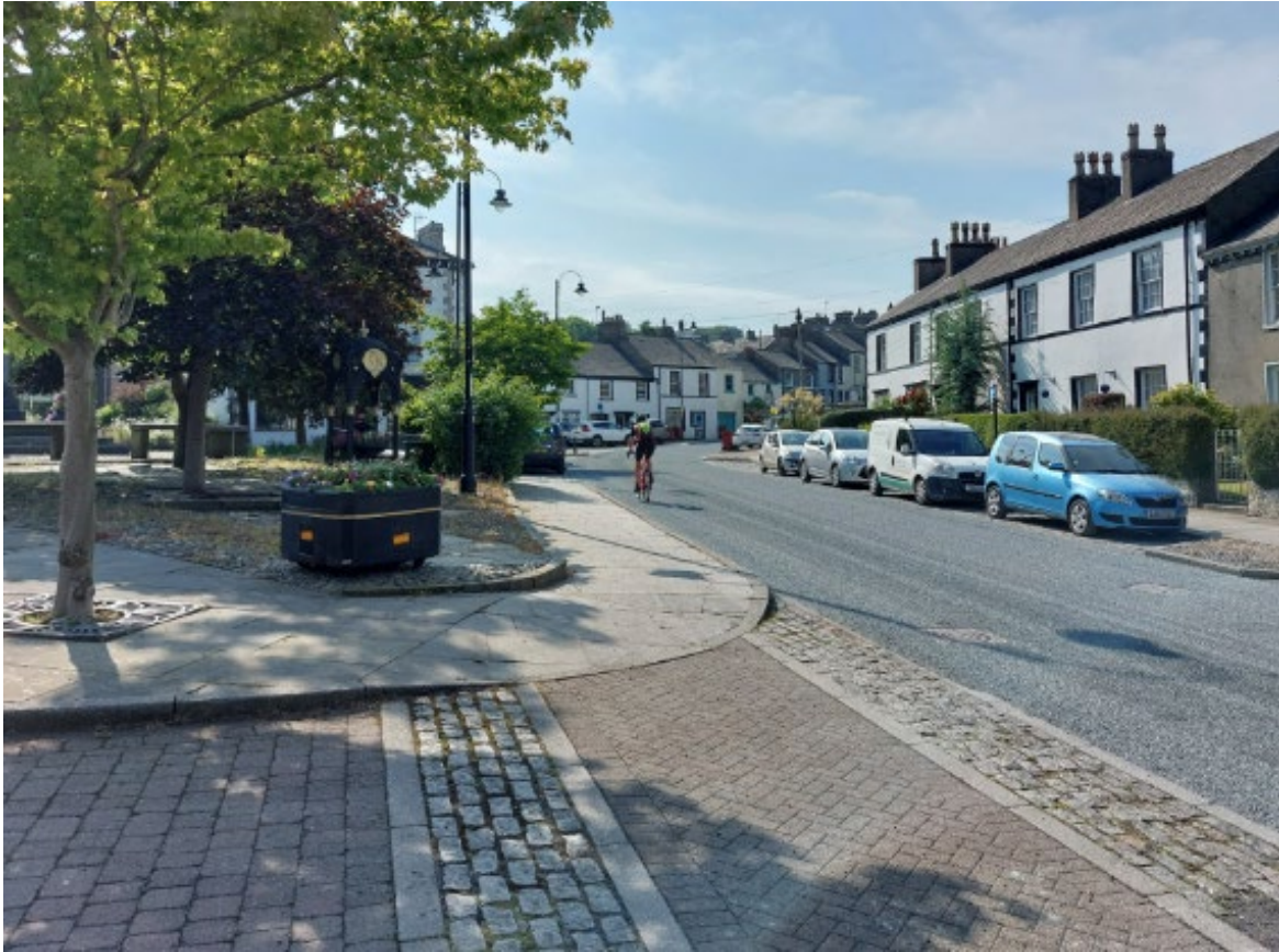
This raised crossing with 'rumble' sets to either side provides a more level crossing for pedestrians and wheelers, slows down vehicles turning into the side streets, and helps to address the priority between motorists and other road users. It forms a coherent and attractive feature in the wider public realm which uses traditional and modern materials. Dalton.
