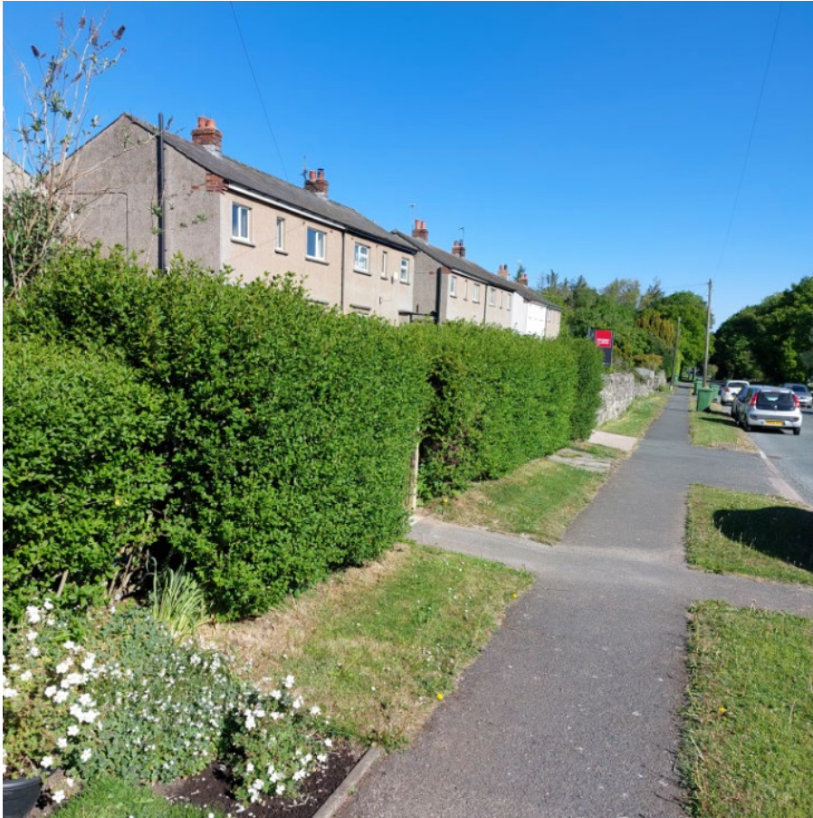
A regular building line of semi-detached houses in Newbiggin. The building line is echoed by the line of the hedges and walls, the verges, pavement and kerb line.
