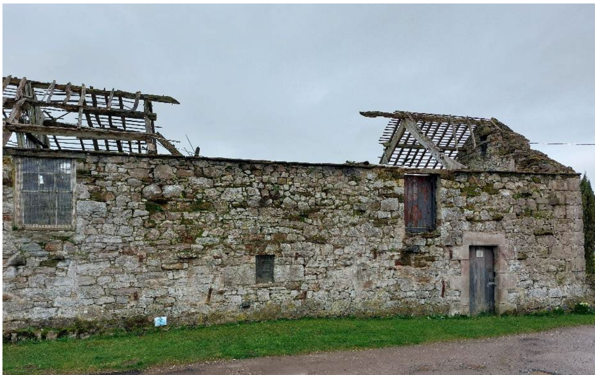
Although derelict, the walls of this barn at Stainton near Penrith are embodied carbon that may be capable of repair, re-use or as a last resort, a source of recycled materials.
