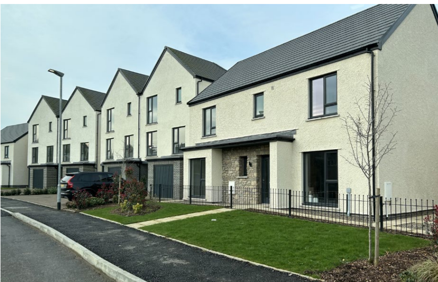
Here, there is a composition of different heights. The central pairs of tall gable-fronted houses are book-ended by two lower broader houses that continue the sweeping building line. Kendal.
