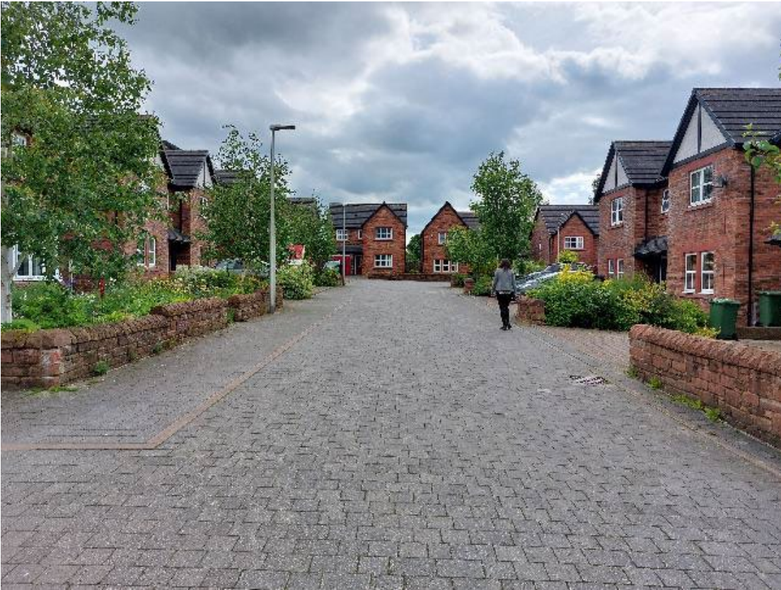
This shared space in Lazonby notionally has a pavement along the left-hand side, but the space is level and shared. This slows motor traffic by subtly making what is normally the carriageway shared by all.
