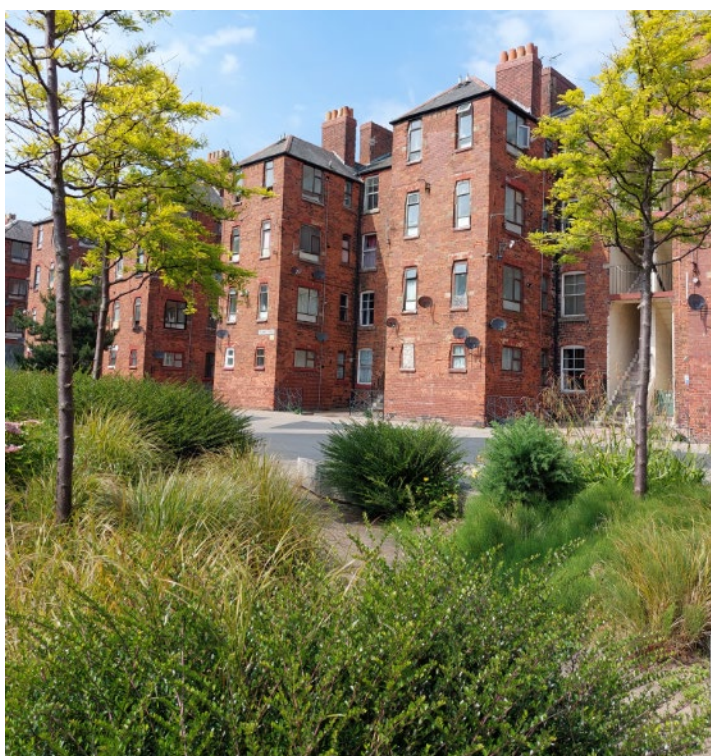
The buildings and highways encourage run-off of rainfall and surface water, but this garden slows it and intercepts it. The garden therefore helps to manage water on the site as well as offer amenity and a better microclimate to the flats. Barrow.
