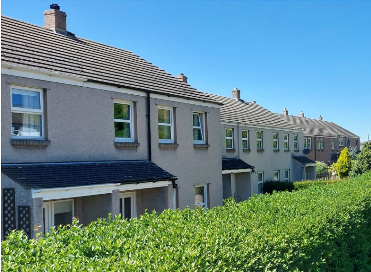
A short row of houses built for social tenants to pattern book designs. Low Hesket.
