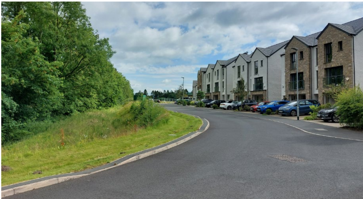
Here in Kirkby Lonsdale, runoff can pass through the dropped kerbs and into a landscaped drainage swale. The swale doubles as amenity landscaping for the houses opposite.
