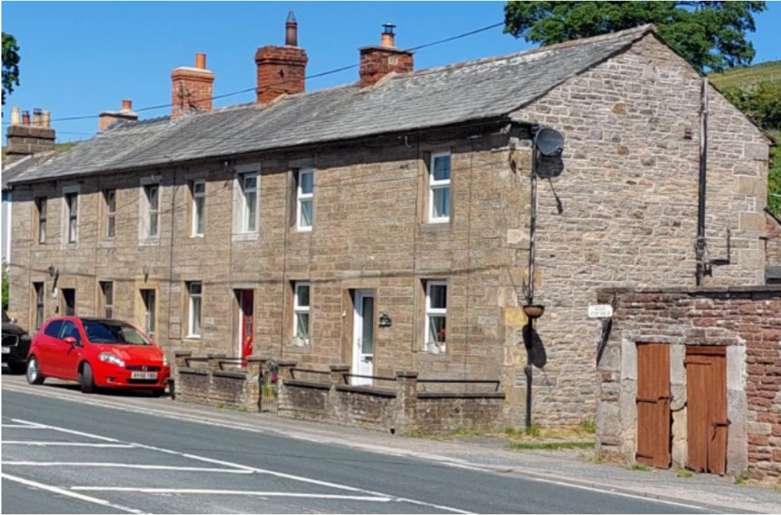
A long or short row of identical or similar houses built for industrial workers. Low Hesket.
