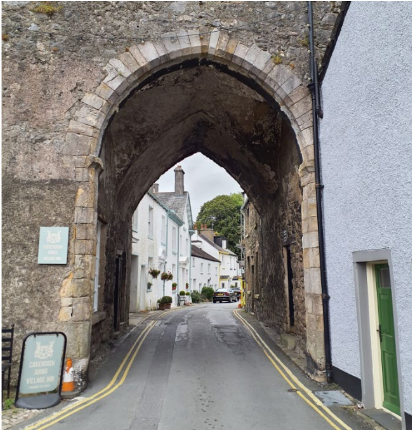
This archway dramatically and physically marks the transition from Cartmel's market place to a much narrower side street. It is these sorts of sudden change and juxtaposition that make places memorable and easy to navigate.
