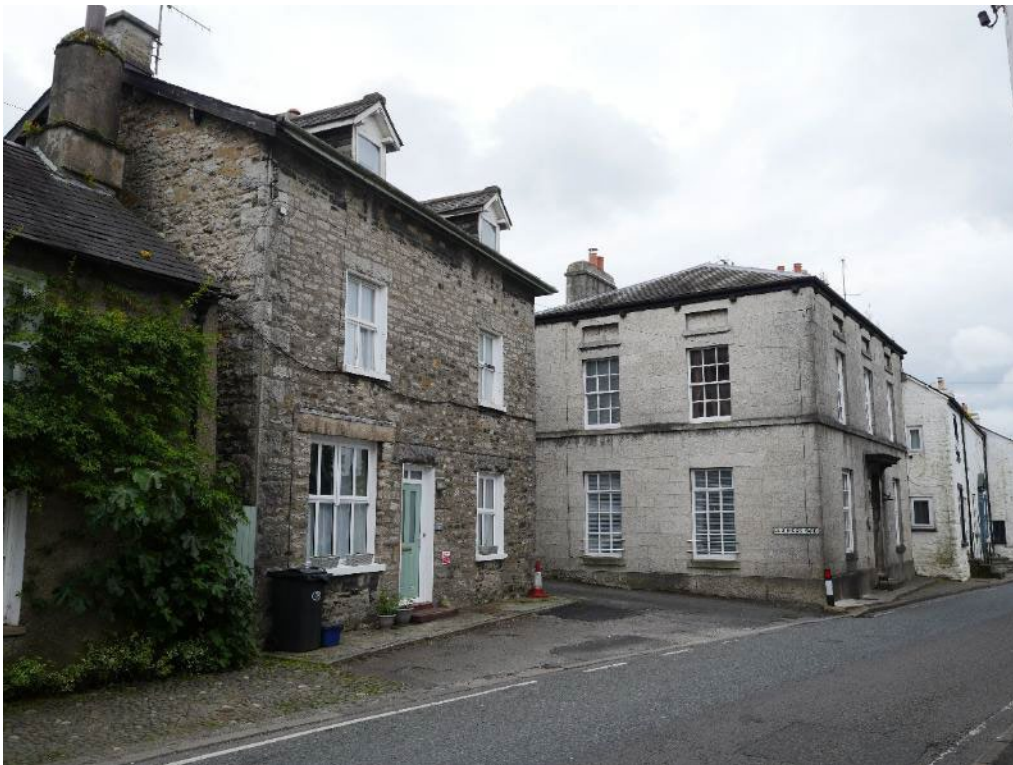
Further up the same street, buildings are possibly oriented for sunlight rather than to face the street, so the building line is a jagged sawtooth-like line with a splayed space between each building and the carriageway. Burton-in-Kendal.
