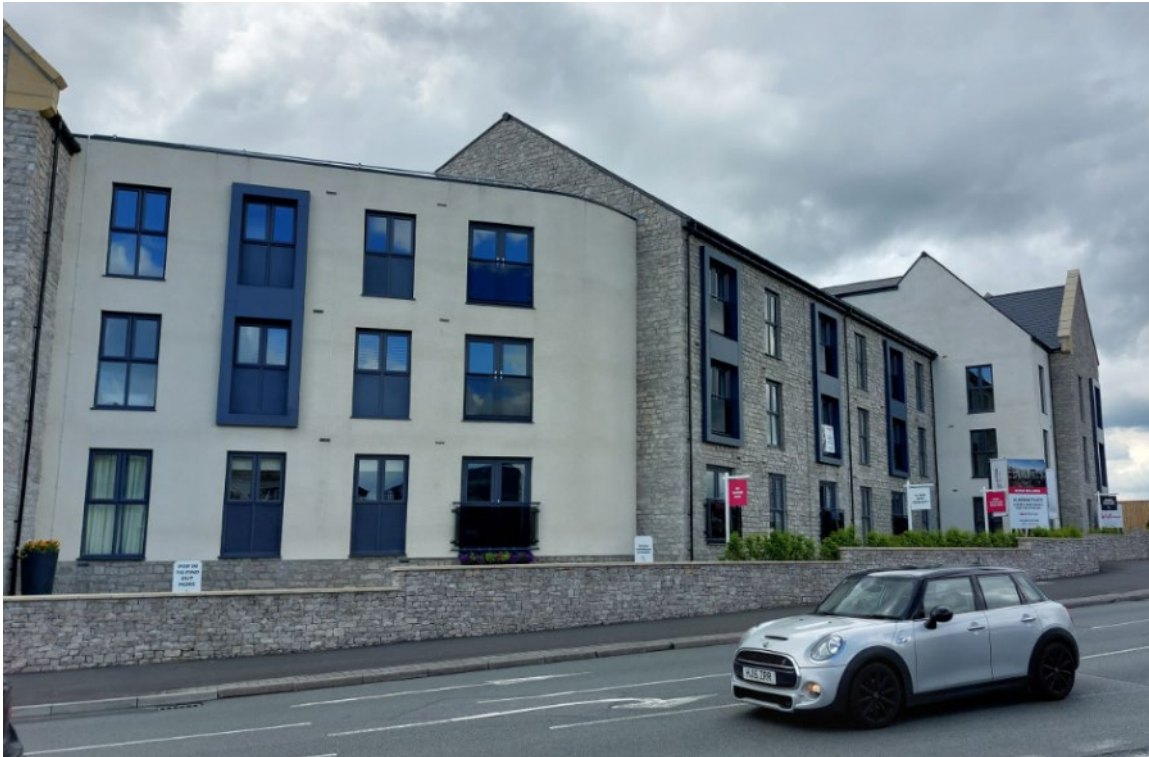
A staggered building line that sweeps around the corner in stages before breaking forward at the far right. This irregular building line helps to break up the mass of a large apartment block in Kendal.
