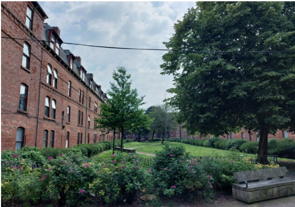
This greenspace provides amenity, access to nature and somewhere to sit or walk. It is shared by residents and is well-overlooked by homes. Barrow.
