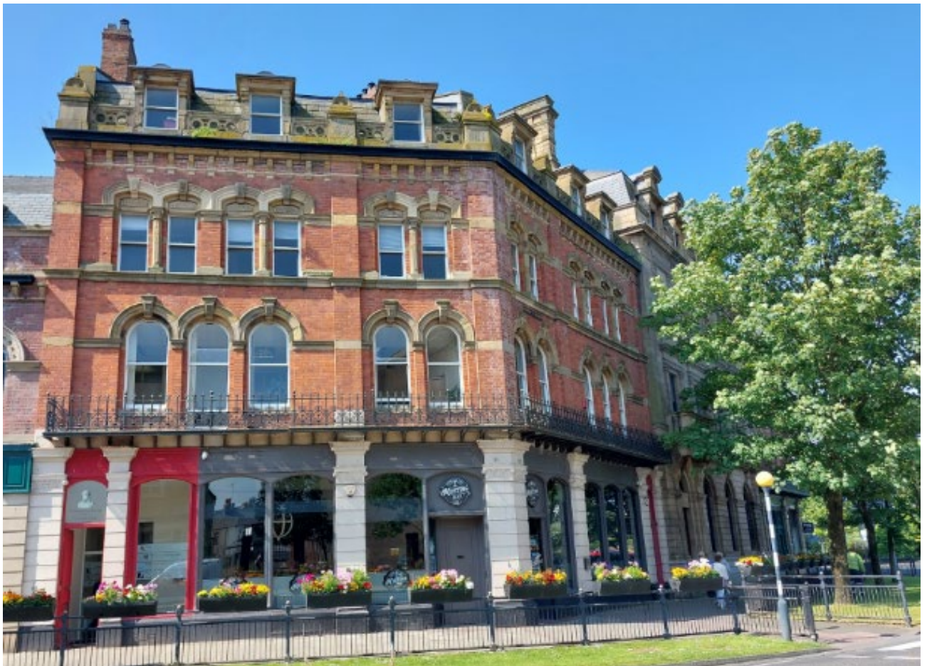
A grand row or crescent of large houses built to a planned layout. Barrow.
