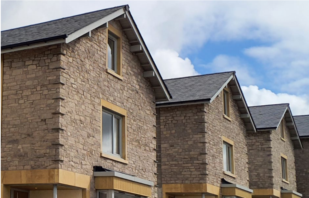
A range of projecting and recessed features – both large and small – add interest and character to these new houses in Lindal-in-Furness
