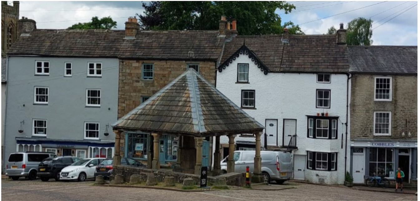
A row of tightly packed buildings of different ages, materials proportions and styles on the narrow building plots lining a market place or commercial street. Alston.
