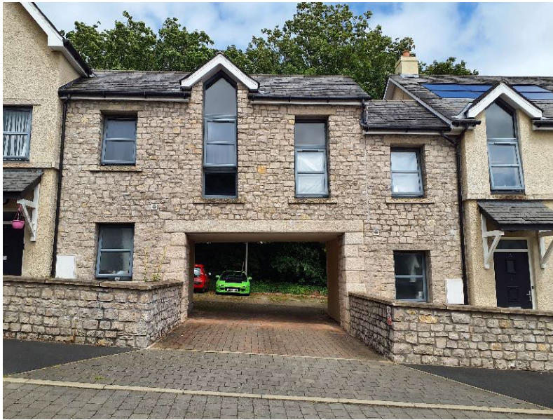
In the same development as the photo above, a concealed courtyard is another means of keeping the street free of parked cars. This in turn enables the street to be more traditional in its width and proportions.
