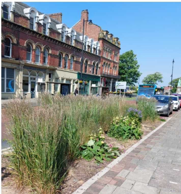
SuDS can be designed-in to new places or retrofitted into existing places. This rain garden in Barrow town centre is a destination for run-off from pavements and buildings, intercepting and slowing the flow of surface water.
