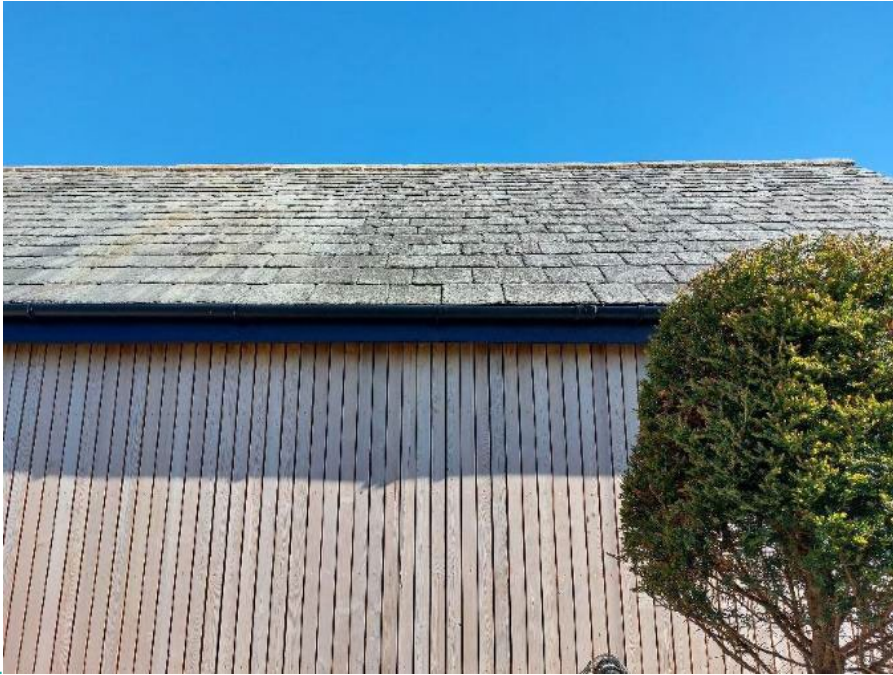
Natural slate and timber have lower embodied energy and can be re-used or recycled. Greystoke.
