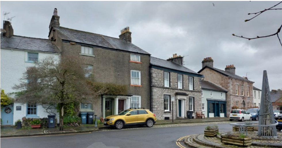
The building ages, types, windows and walling material, and colours all vary along this row, but the roofs are all slate, gabled and vary only slightly in their pitch. The roofs and accents provided by the chimneys help to unify the row. It also shows how tried and tested methods and forms of building persisted even as fashions changed. Ulverston town centre.
