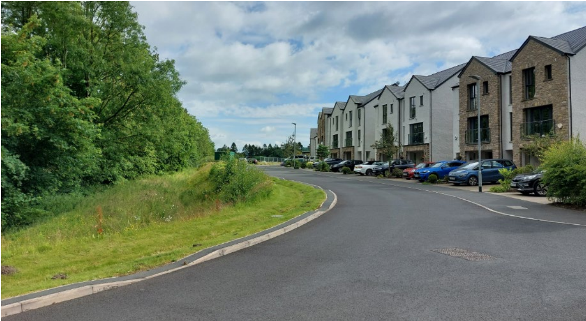
Here in Kirkby Lonsdale, runoff can pass through the dropped kerbs and into a landscaped drainage swale. The swale doubles as amenity landscaping for the houses opposite.
