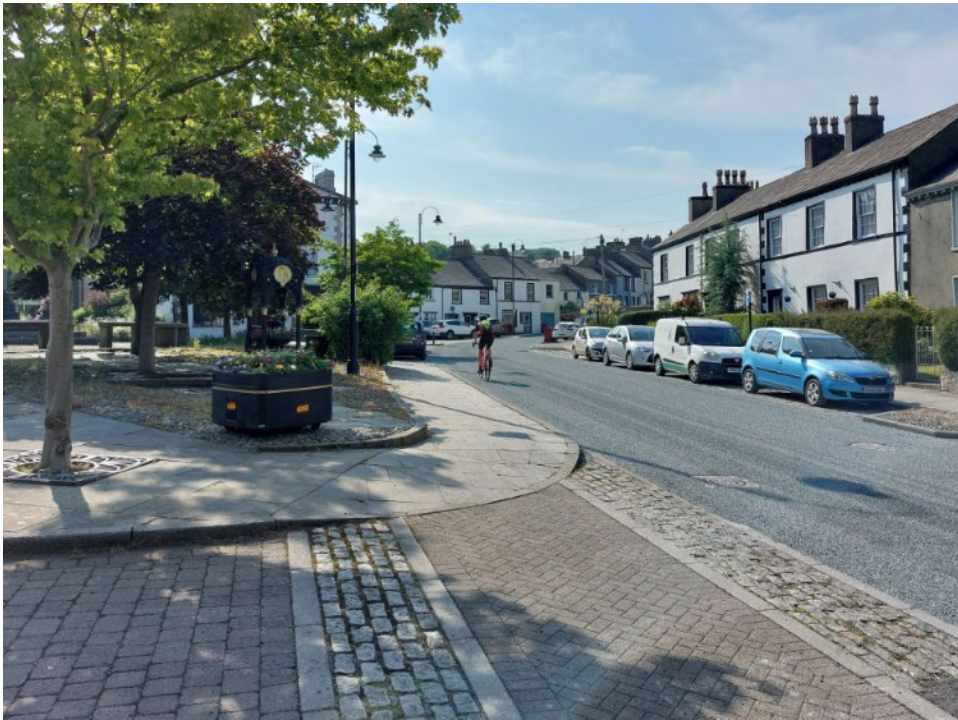
This raised crossing with 'rumble' sets to either side provides a more level crossing for pedestrians and wheelers, slows down vehicles turning into the side streets, and helps to address the priority between motorists and other road users. It forms a coherent and attractive feature in the wider public realm which uses traditional and modern materials Dalton.
