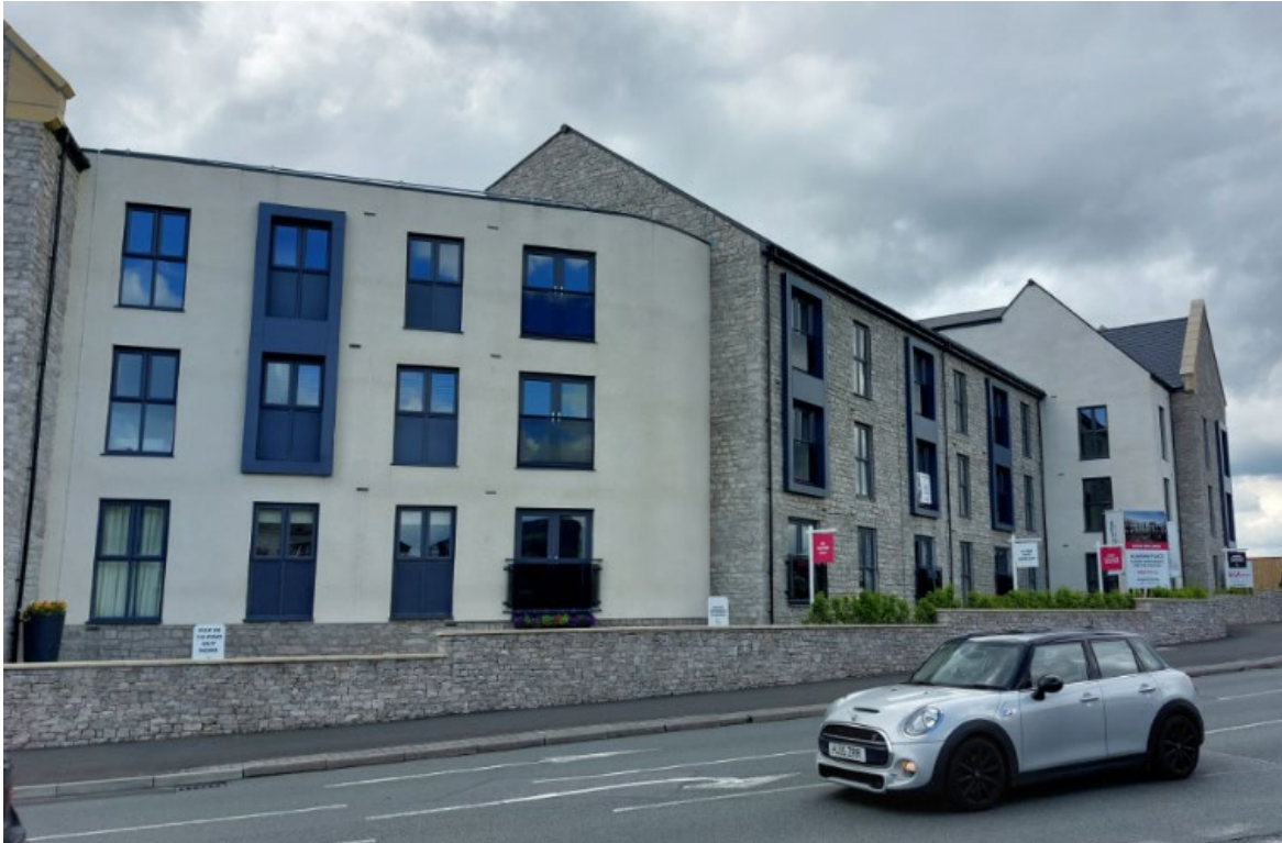
A staggered building line that sweeps around the corner in stages before breaking forward at the far right. This irregular building line helps to break up the mass of a large apartment block in Kendal.
