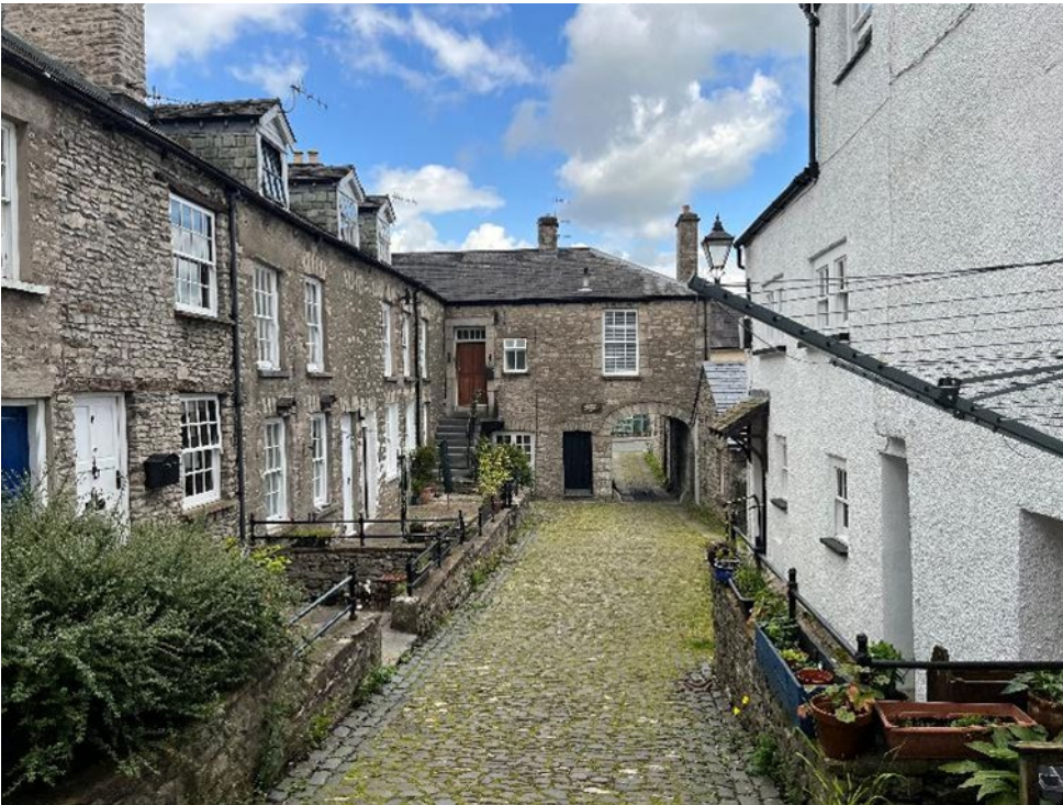
The district's market towns have a shared tradition of yards that link two larger streets but have a much more intimate character due to their widths and degree of overlooking by homes. Other than providing a shortcut for pedestrians, they have a sense of privacy and community. Kendal.
