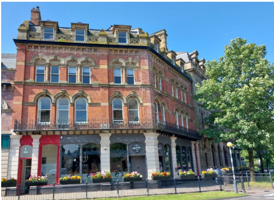
A grand row or crescent of large houses built to a planned layout. Barrow.
