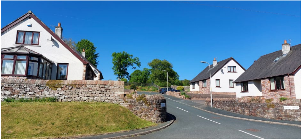
The retention of stone walls and re-use of the walling stone are a good re-use of embodied carbon on the site, as well as knitting the development into the character of Greystoke.
