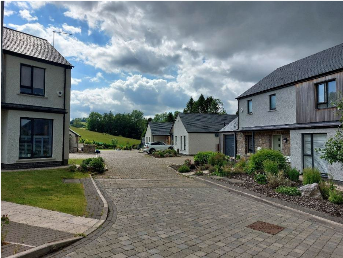
Views out to the countryside enhance the design and character of any housing development. These views provide a crucial link to place and context and add a different dimension to the street scene. Kirkby Lonsdale.
