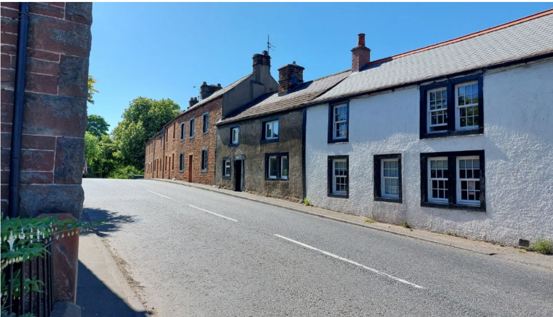
Bare stone, natural colour render and painted render side by side, giving a variety of textures along with the variations in the designs of the houses and cottages. Langwathby.
