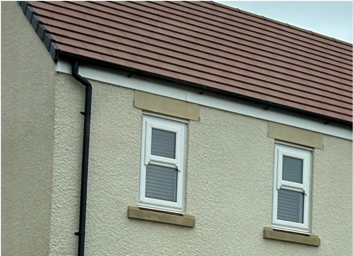
The exterior of this new house is entirely made of materials that are energy intensive (artificial stone sills and lintels and synthetic / cement render) or have short lifespans and will go to landfill (uPVC rainwater goods, fascias and windows). Penrith.
