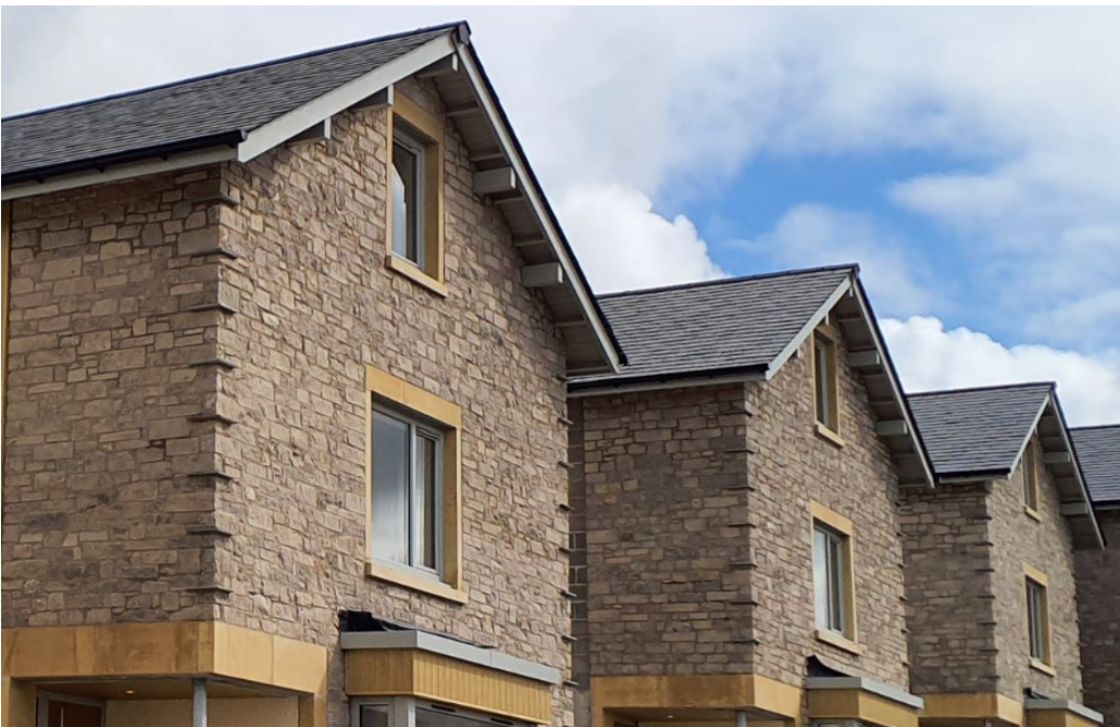
A range of projecting and recessed features – both large and small – add interest and character to these new houses in Lindal-in-Furness
