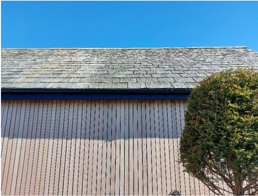
Natural slate and timber have lower embodied energy and can be re-used or recycled. Greystoke.
