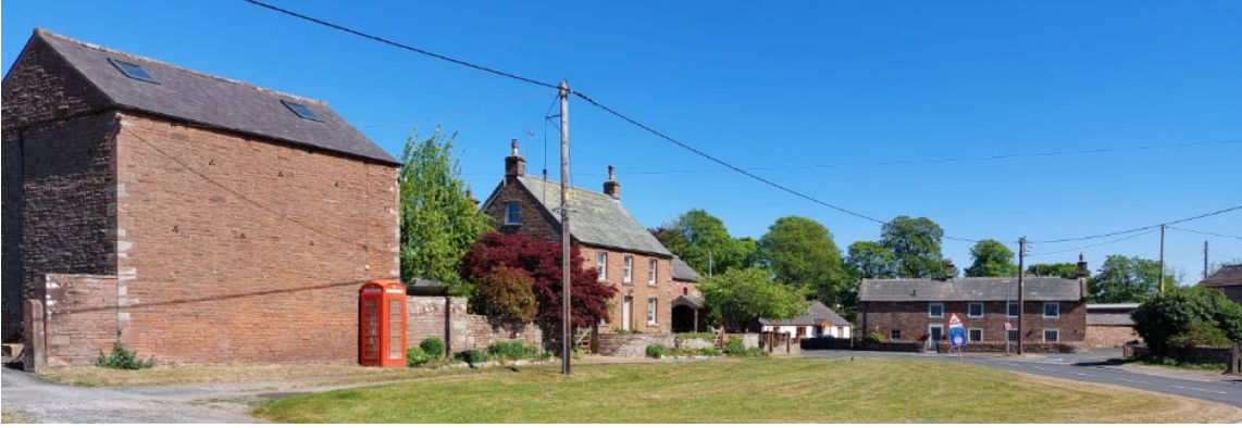
Three very different buildings achieve harmony through the use of similar local stone and a mix of local and Welsh slate. Langwathby.
