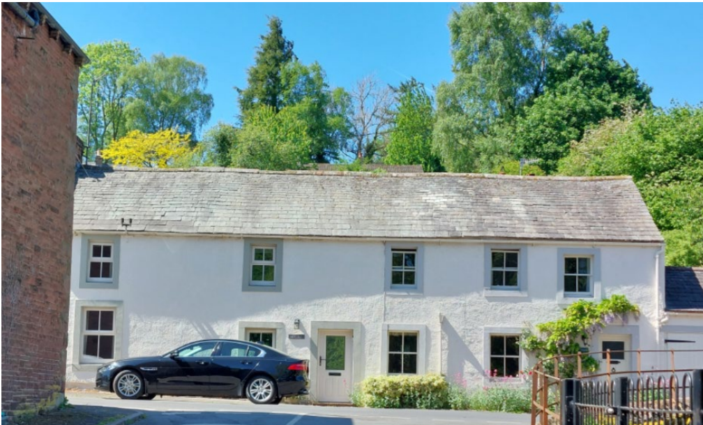
A house facing directly onto the street and having a positive presence in the street scene. Armathwaite.
