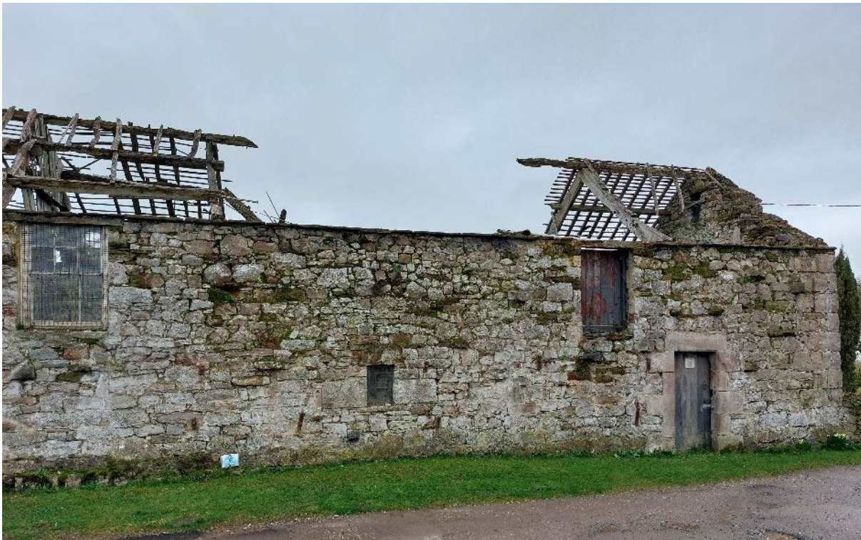
Although derelict, the walls of this barn at Stainton near Penrith are embodied carbon that may be capable of repair, and re-use or as a last resort, a source of recycled materials.
