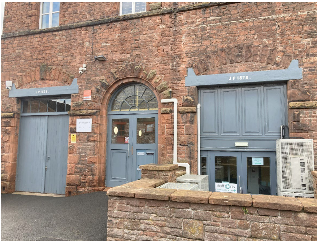
The historic masonry openings have been kept and re-purposed in different ways to suit the mill's new use.
