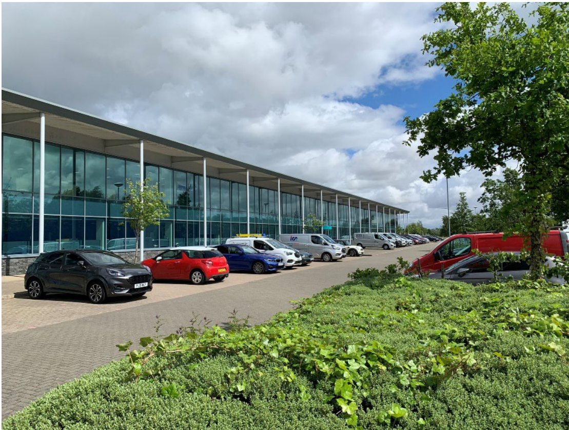
The quality of this development is lifted by a few simple measures: space given for a range of planting, including trees; the use of natural colours in the permeable modular paving rather than bitmac; and the deep shading of the expanses of glass. The building itself is simple yet elegant, the glazing reflecting the sky and trees, and resting on a shallow slatestone plinth. Ulverston.
