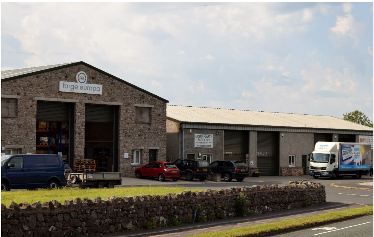
The use of stone cladding and roughcast render give this modern business development a local and rural character. The use of stone and render in different ways suggests a hierarchy of buildings, which is reinforced by the layouts of the openings. The broad gabled forms and corrugated roofs also recall modern farm buildings. The local materials complement the retained stone boundary wall in the foreground. Dalton.
