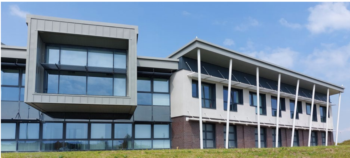
At this business park in Barrow, the glazing maximises daylight but reduces glare and overheating by using recessed glazing and shades over glass.
