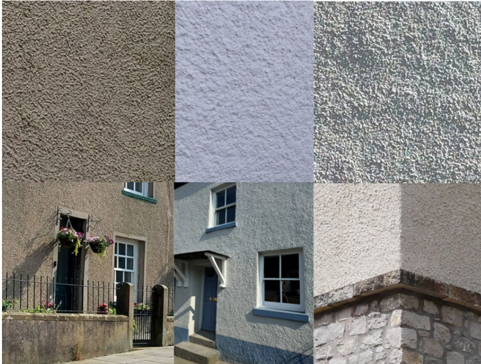
The six examples above are from different towns and villages in Westmorland and Furness: Ulverston, Kirkby Lonsdale, Langwathby, Grange-over-Sands and two examples in Dalton: painted and natural.
