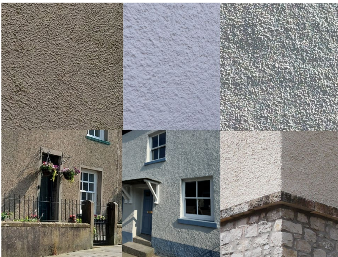
These examples of roughcast render are from different towns and villages in Westmorland and Furness: Ulverston, Kirkby Lonsdale, Langwathby, Grange-over-Sands and two examples in Dalton, painted and natural.
