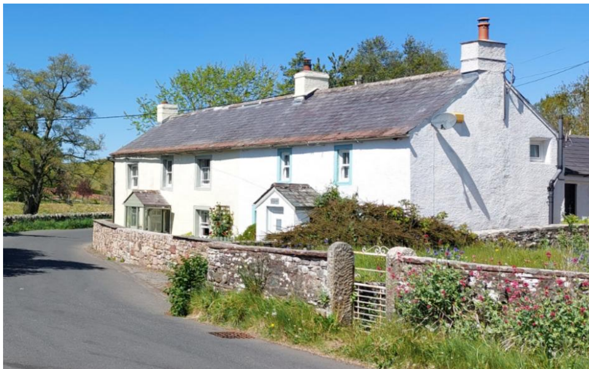
Millhouse borders the Lake District, and this is evident in the Cumbrian blue slate roof with distinctive stone slate lower course and the smaller openings and extra-solid looking walls. These minor variations within the materials and design of buildings across the district must not be lost through the use of generic details or standard materials and details.
