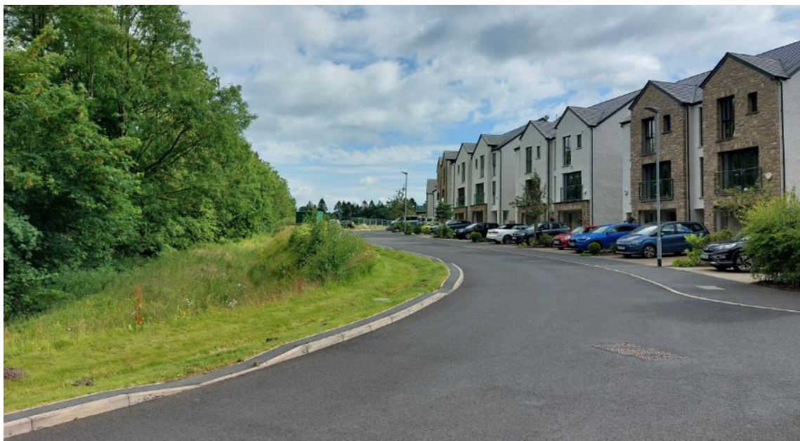
Here in Kirkby Lonsdale, runoff can pass through the dropped kerbs and into a landscaped drainage swale. The swale doubles as amenity landscaping for the buildings opposite.
