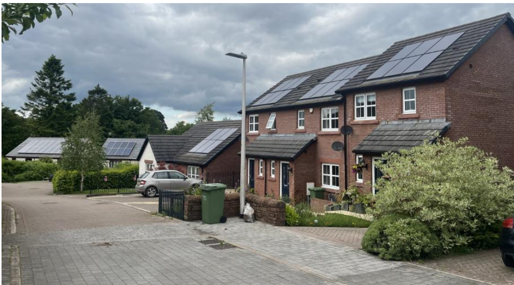
PV panels have been built into the roof slopes in the foreground when these buildings were built, meaning the surfaces of the panels are almost flush with the roof tiles. In the background PV panels have been retrofitted to existing slate roofs. Lazonby.
