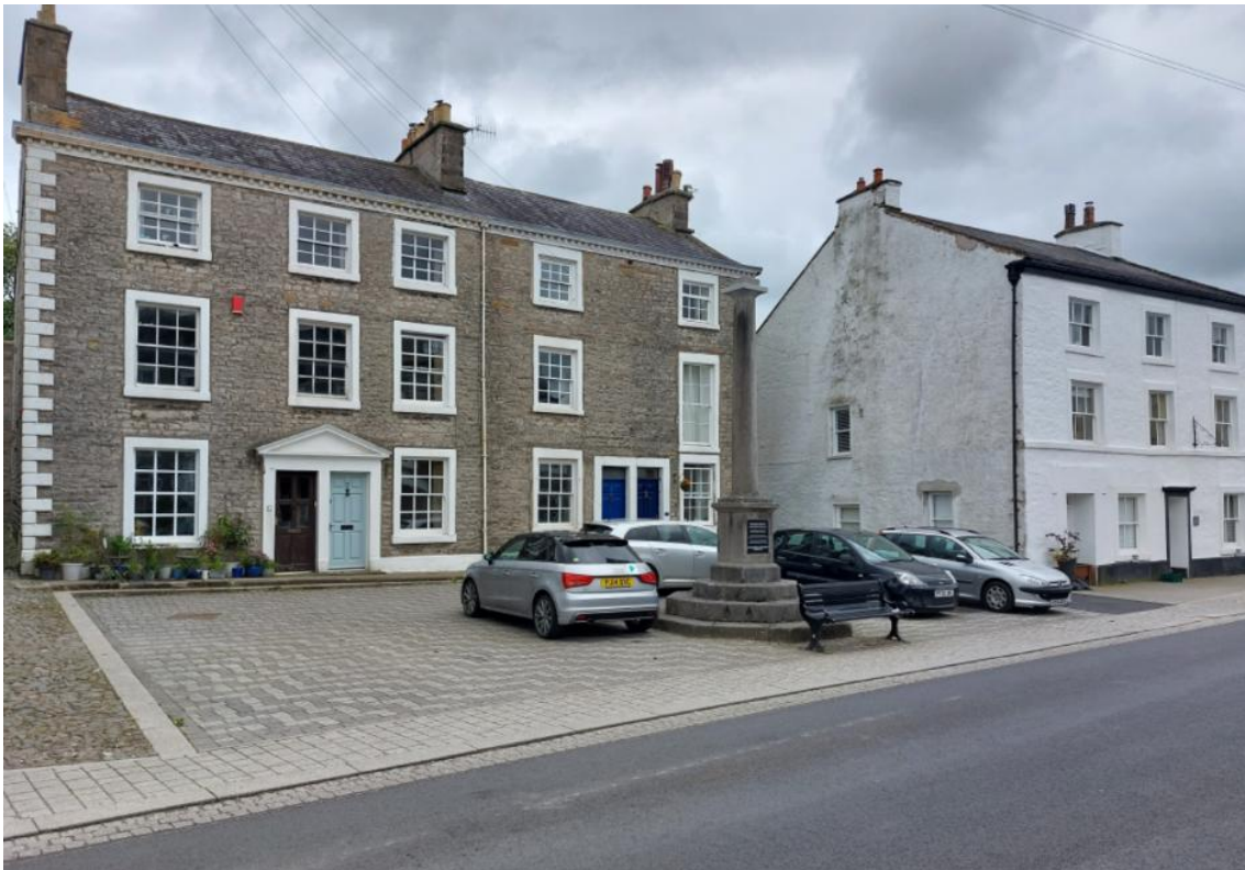
This small area of public realm in Burton-in-Kendal has day-to-day use as informal parking, but its flexible design means it could easily be used on occasion for small community events or gatherings, and the cars park elsewhere.
