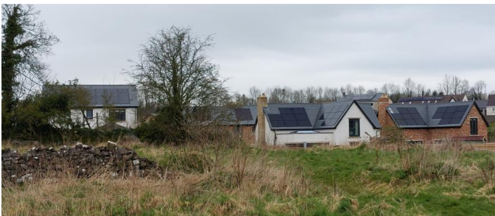
This development in Stainton near Penrith makes extensive use of solar panels on the southerly facing roof pitches. The panels are set into the roof slopes.
