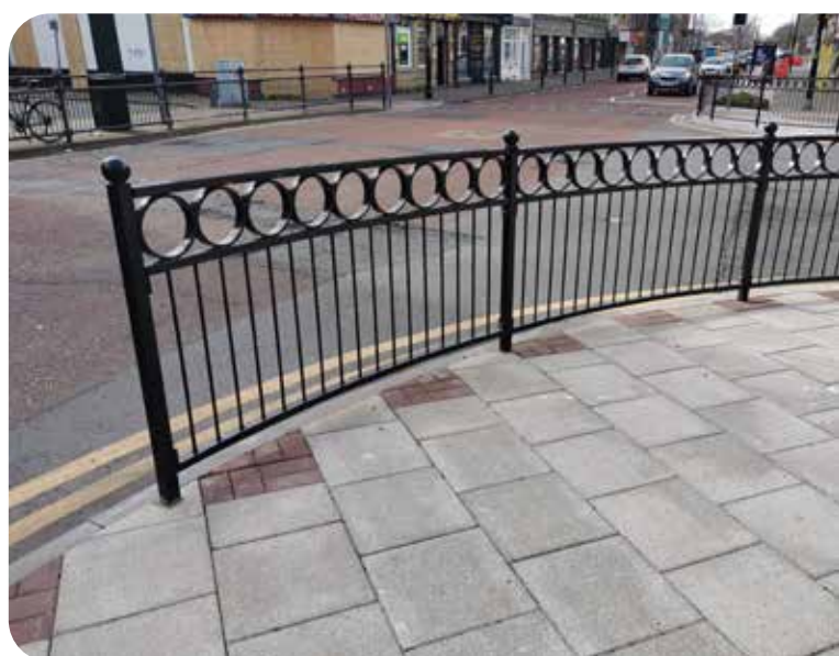
Heritage-style Railings on Duke Street
