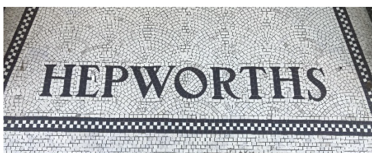
Figure 12 Tiled entrance to shop
