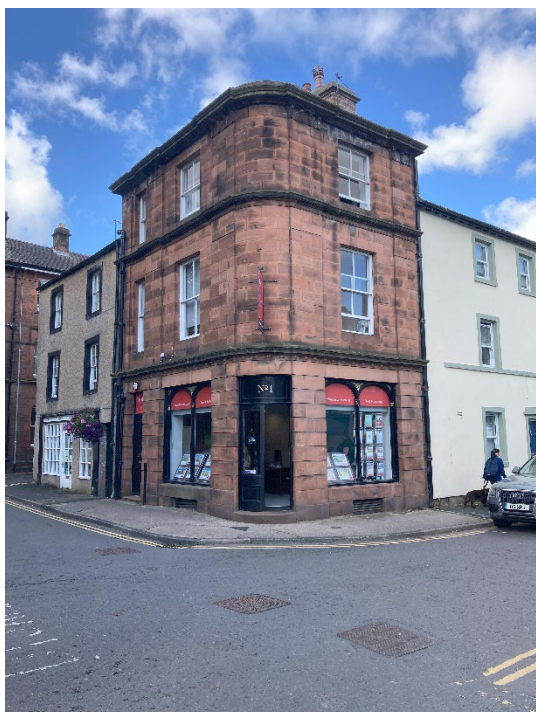
Figure 16 Building line follows street corner
